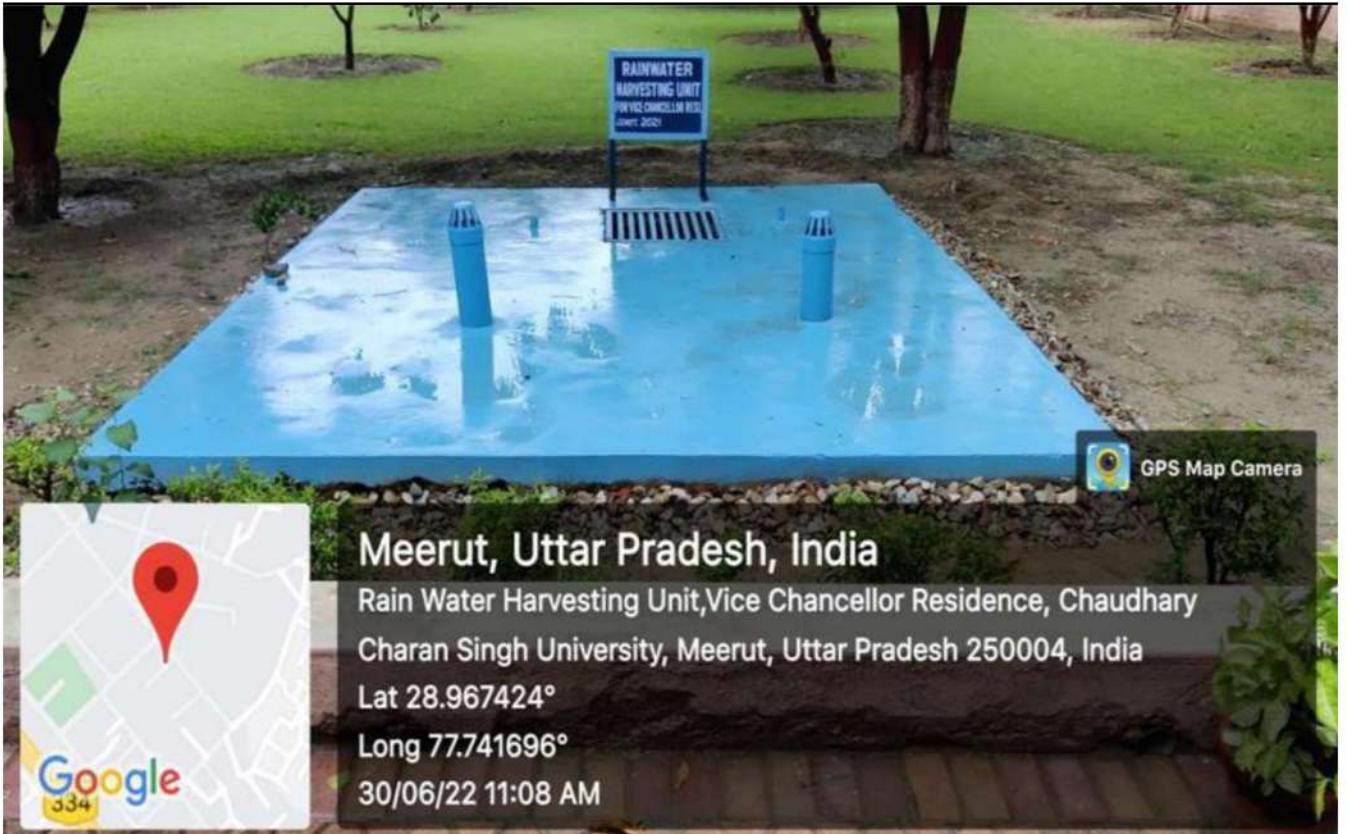
Rain Water Harvesting Unit for V.C. Resi.
