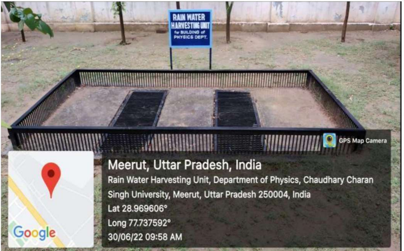
Rain Water Harvesting Units For Dept. of Physics
