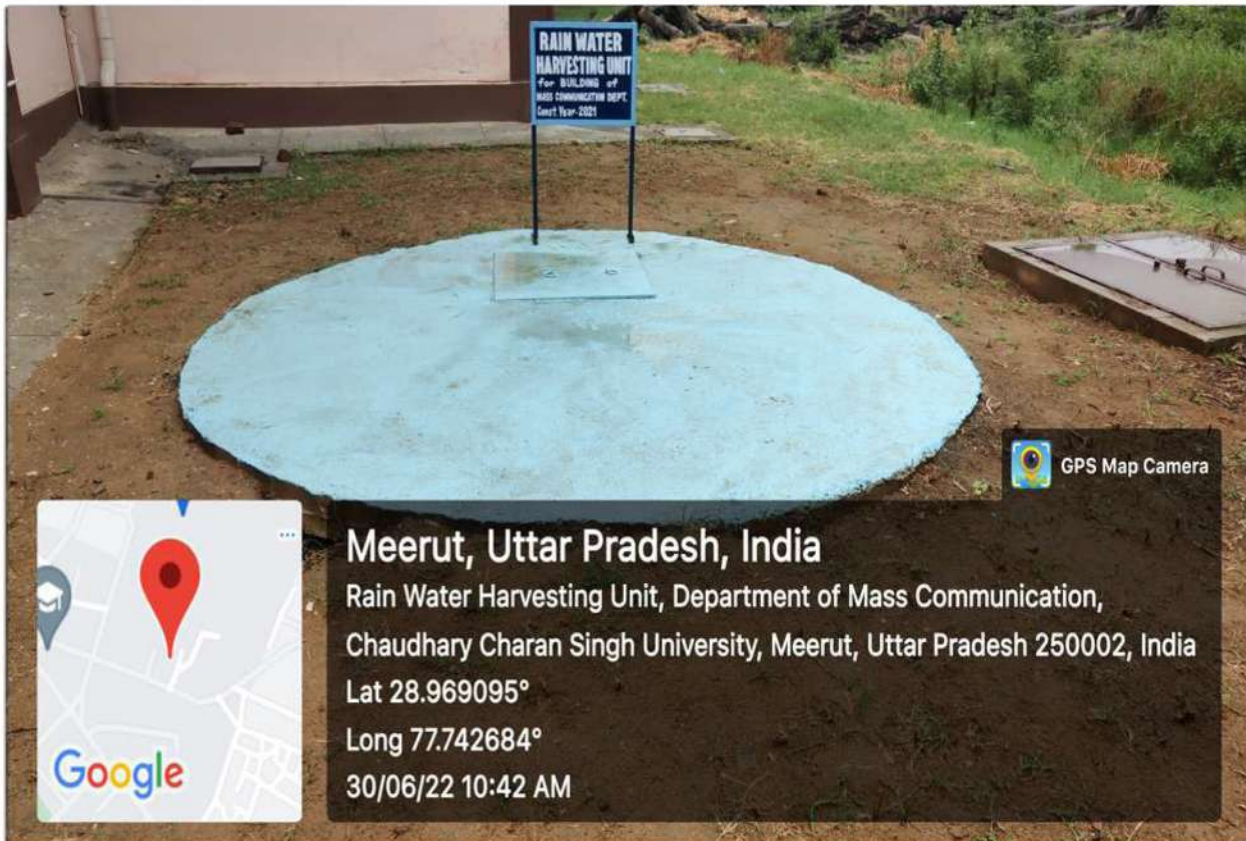
Rain Water Harvesting Units For Mass Communication Building
