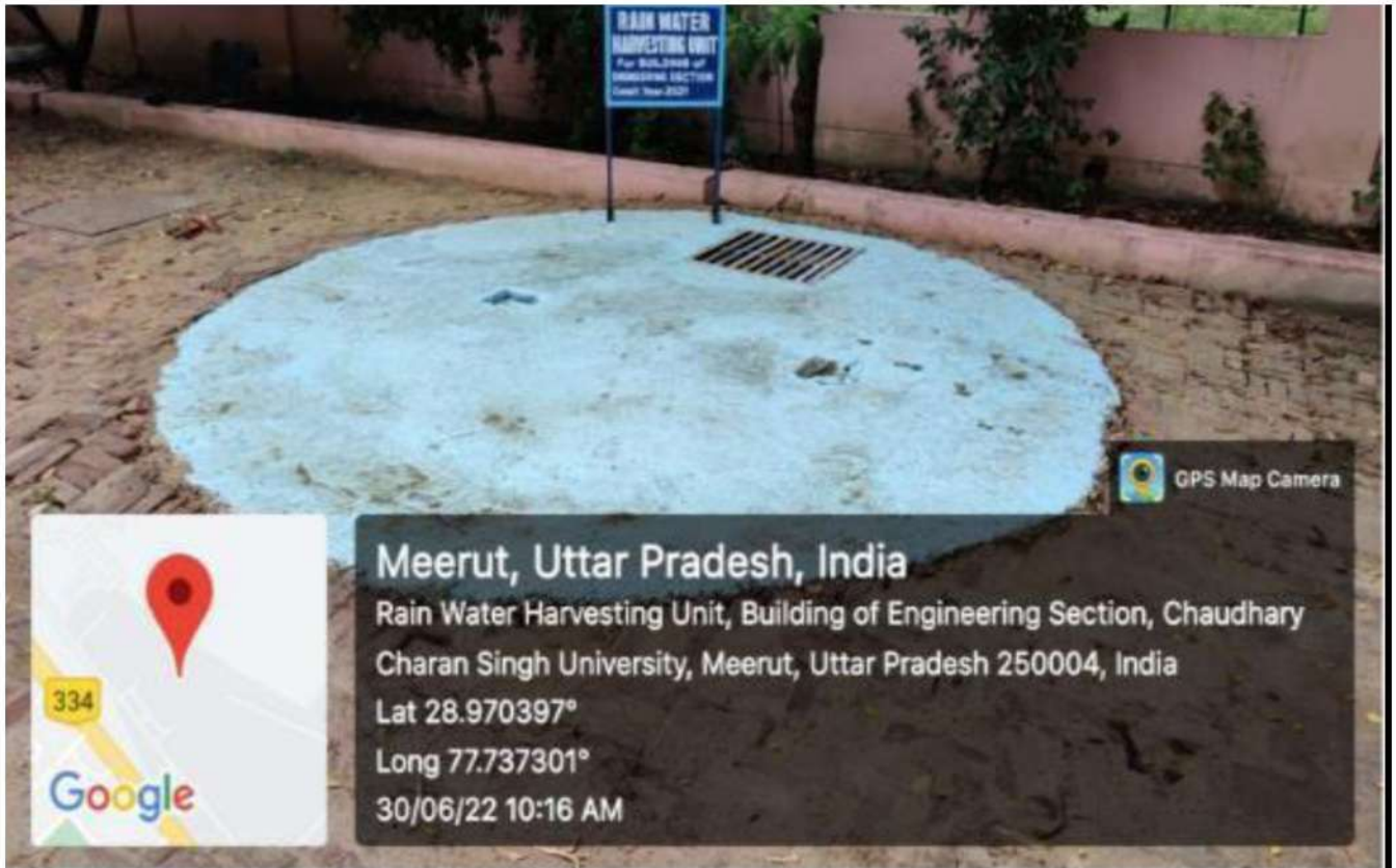
Rain Water Harvesting Units For Engineering Section
