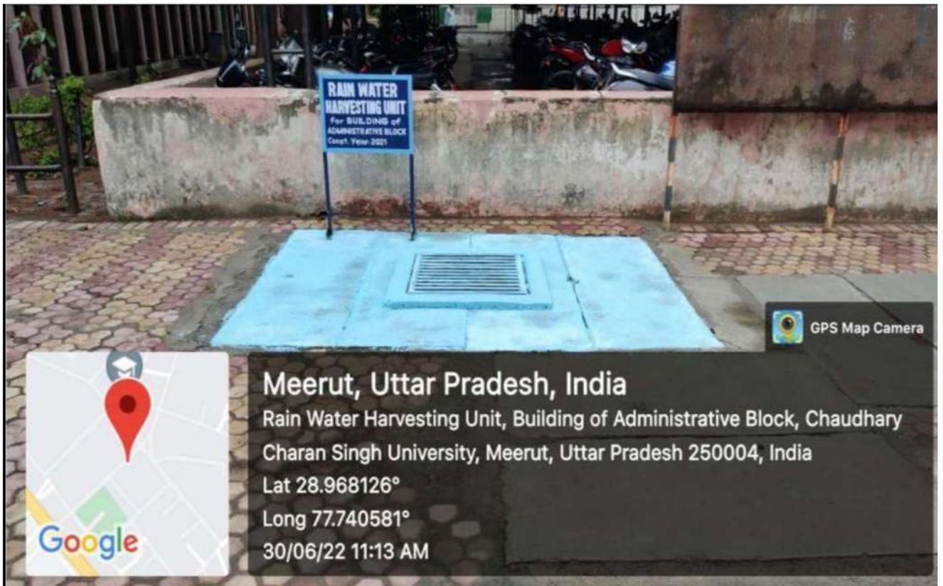
Rain Water Harvesting Unit for Administration Block
