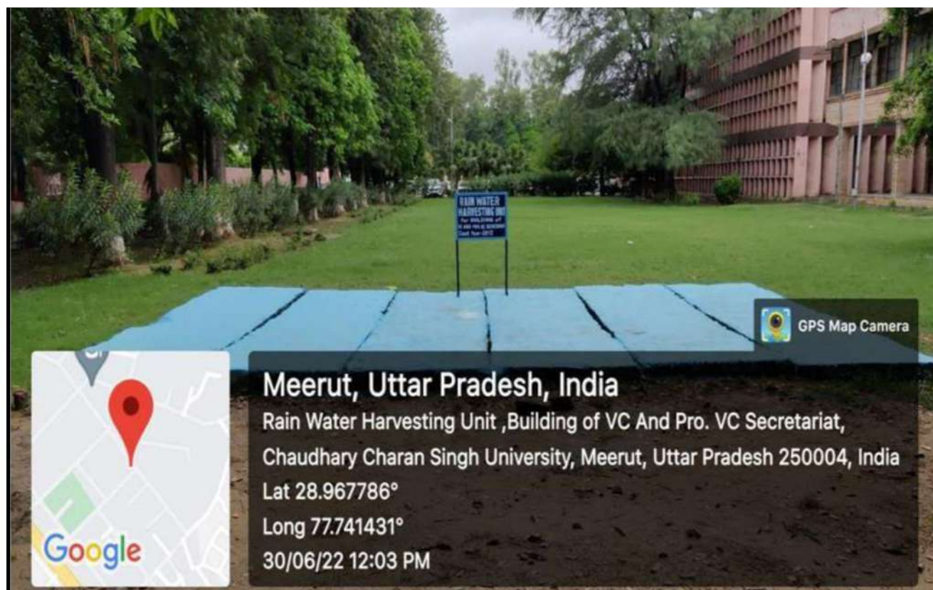
Rain Water Harvesting Unit for Buliding of V.C. & Pro. V.C. Secratarariat
