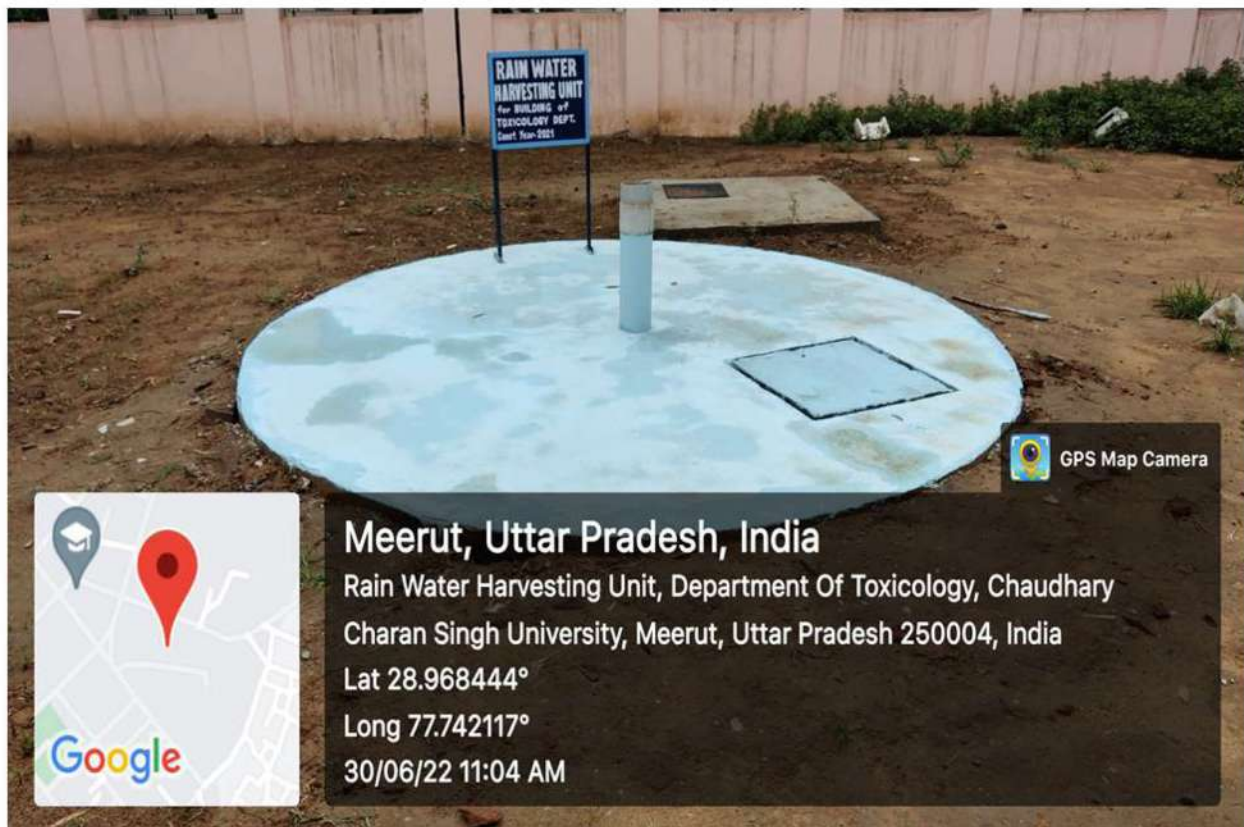
Rain Water Harvesting Units For Toxicology Building
