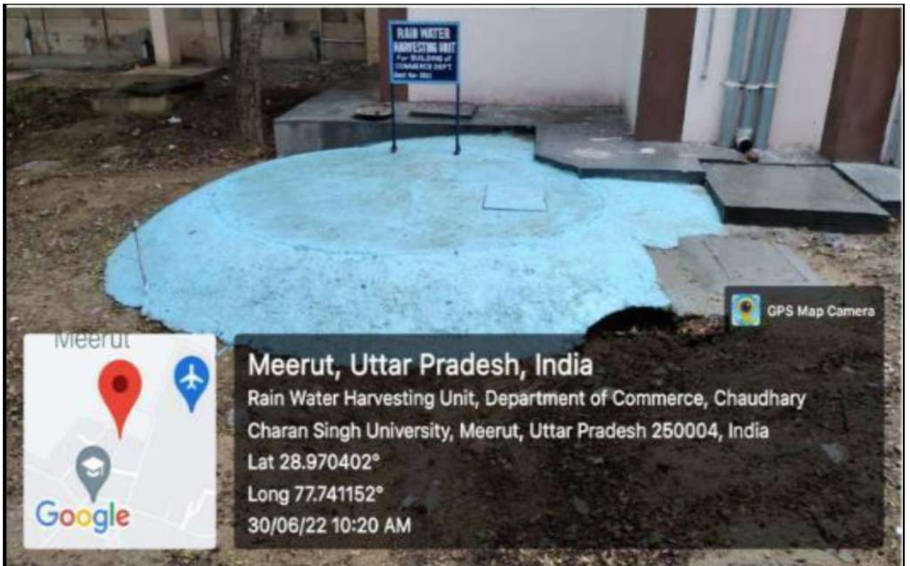
Rain Water Harvesting Unit for Dept. of Commerce
